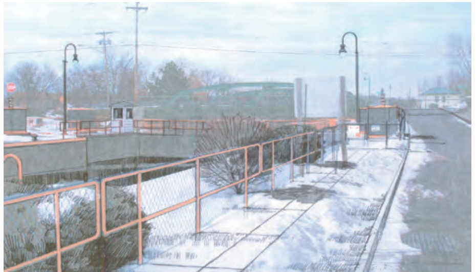
Chain-link fencing on Water Street is replaced with canal-theme railings.
