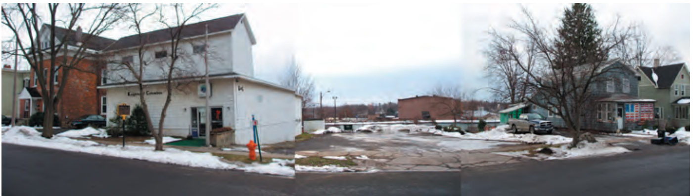
Existing conditions of the Knights of Columbus property
