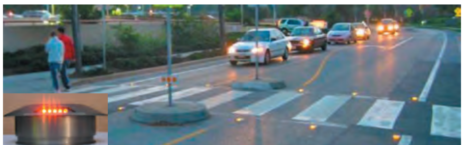
Consider lighted crosswalks at the Four Corner area.
